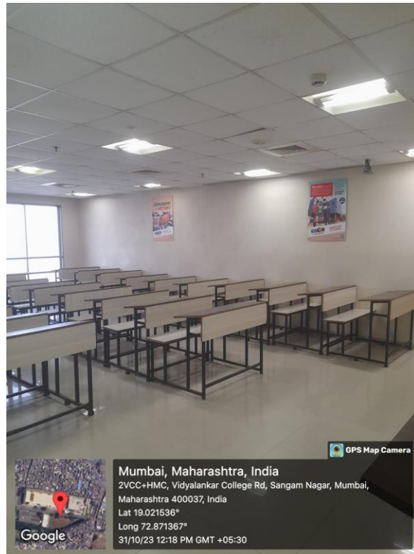
Figure 3.3. LED lights in Classrooms, M-block, VIT
