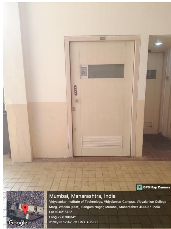
Figure 3.1. Signage boards on Washrooms, VIT
